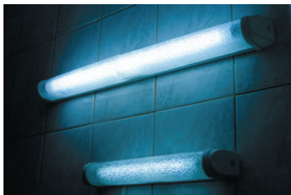
Figure 30.7 These fluorescent light tubes are wired in series with an inductor, or ballast, that helps to sustain the current flowing through the tubes.
