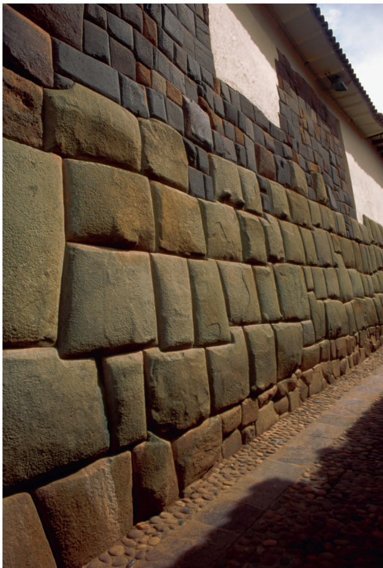
INCA STONEMWORK. In the former Inca capital, Cuzco, Peru, the Spaniards incorporated these earthquake-resistant foundations into their own buildings. © Jeremy Horner/Corbis .
