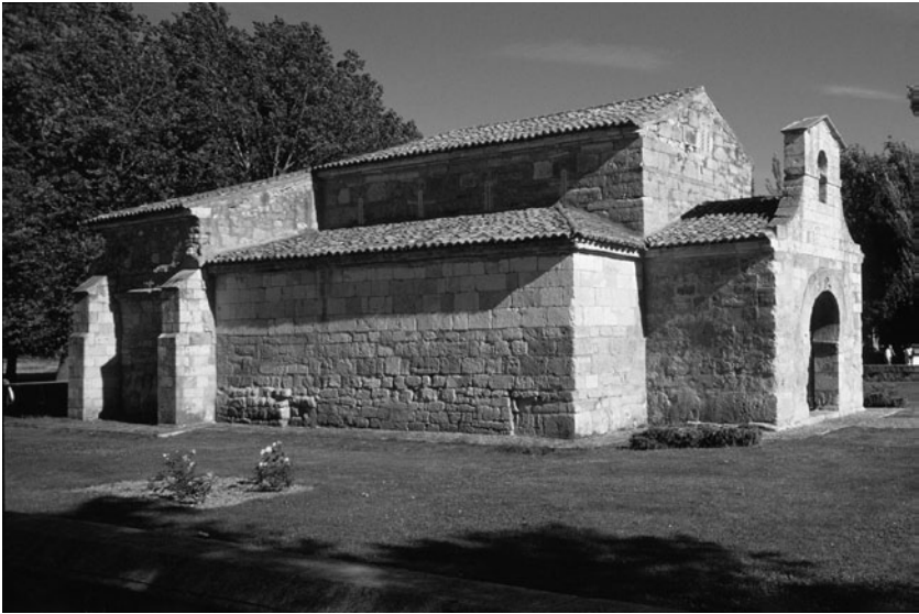
Plate 2 Church of St Juan de Baños, Spain, dedicated in 661
