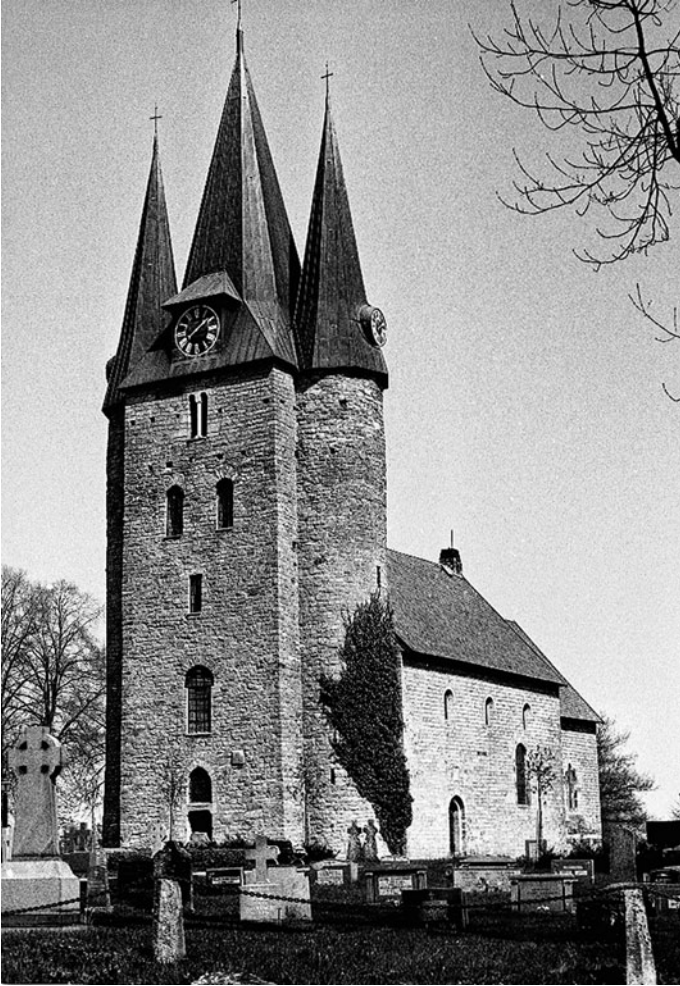
2 Husaby Church, Västergötland. One of Sweden's oldest churches dating from the eleventh century. Its massive tower, with round arched windows, was originally attached to a wooden nave which was replaced in the following century by a stone nave and choir. Its style is Romanesque, largely derived from models in the German Rhineland typical of stone churches built in Sweden at this time. Photo: Anna Nilsén.
