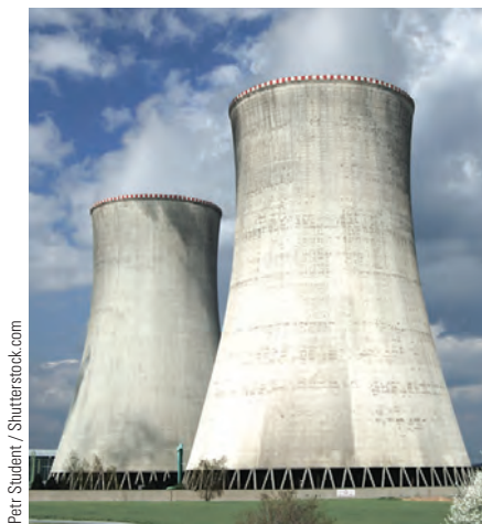
(b) Nuclear reactors have cooling towers in the shape of hyperboloids.
