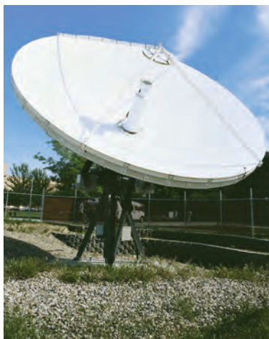
(a) A satellite dish reflects signals to the focus of a paraboloid.
