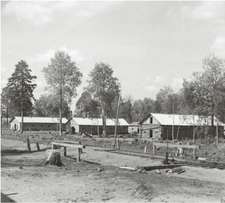
Building the railway to Murmansk across the Kola peninsula, 1915.
