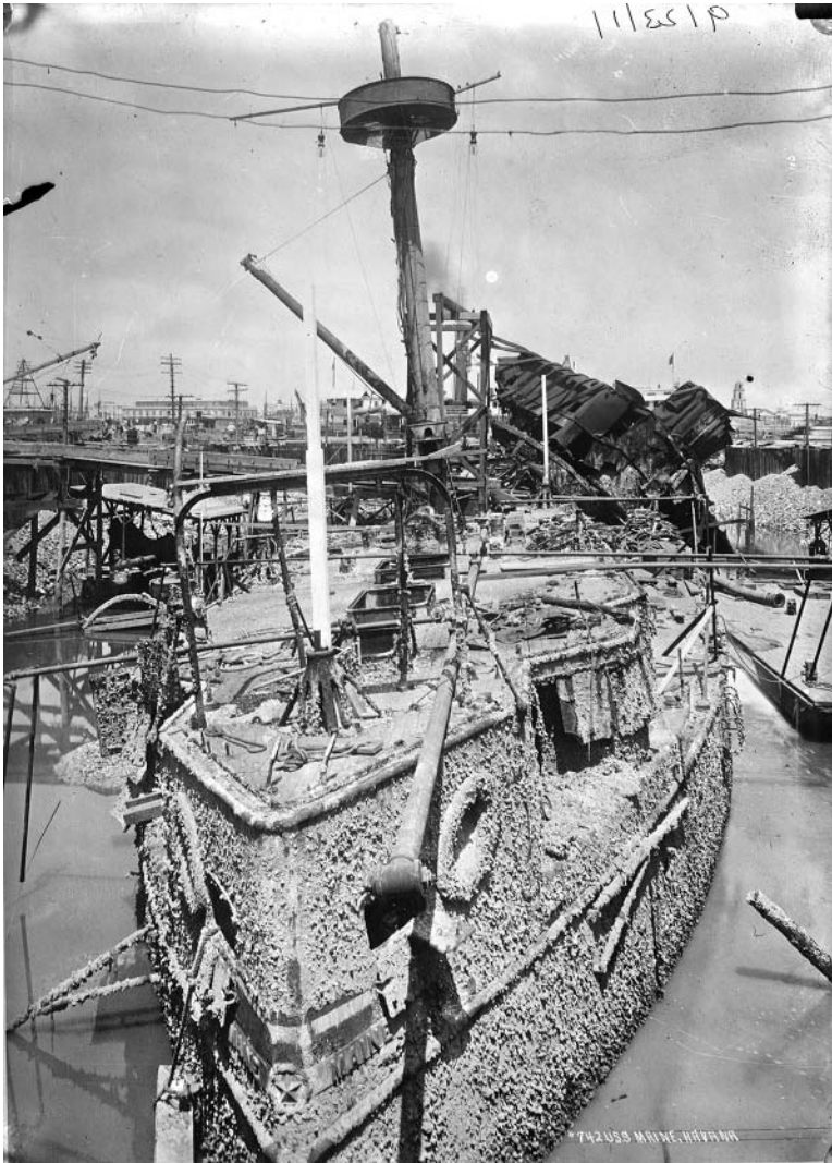
USS Maine , Havana, September 23, 1911. In 1910 the US Congress directed the secretary of war and the chief of engineers to raise the wreck from Havana harbor and instructed that the remaining bodies be buried in Arlington National Cemetery. (Library of Congress Prints and Photographs Division, Washington, DC)
