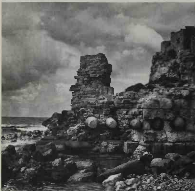
Roman columns built into the Crusader masonry at Caesarea, then the Roman provincial capital, port and military base.
